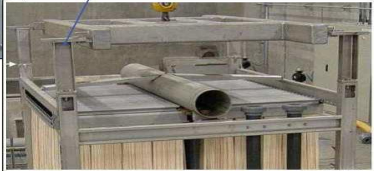
Install Hanger Arm Extensions (provided by GE-ZENON)
